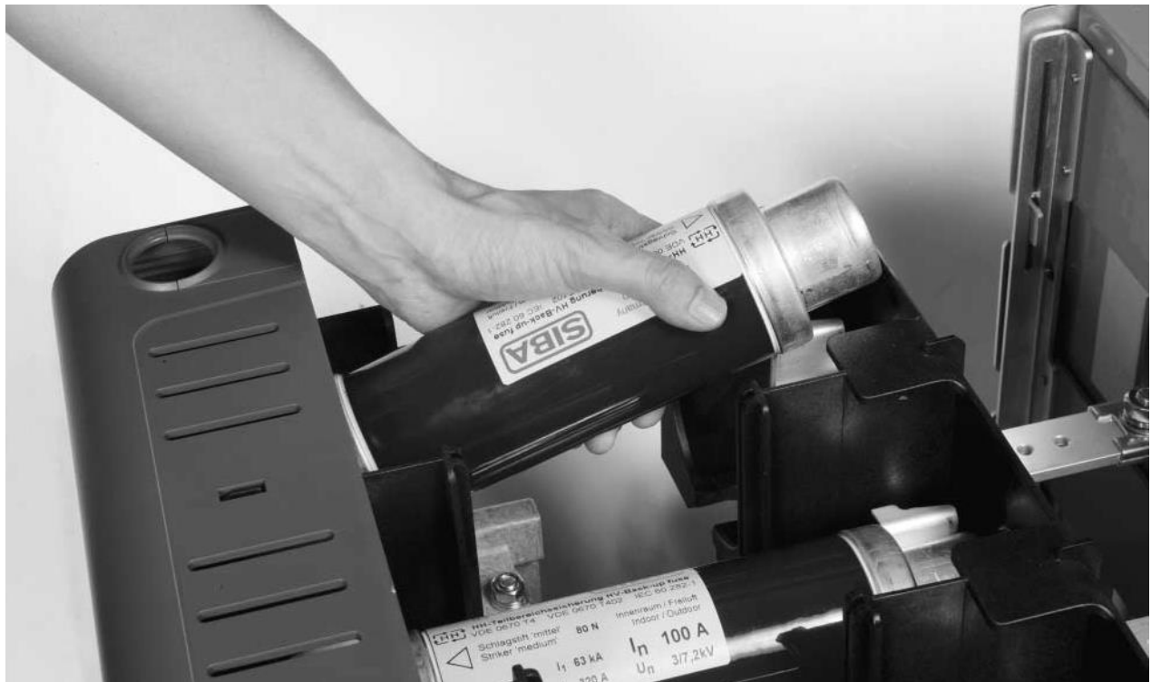
Fig. 4.2 Replacing the fuse
